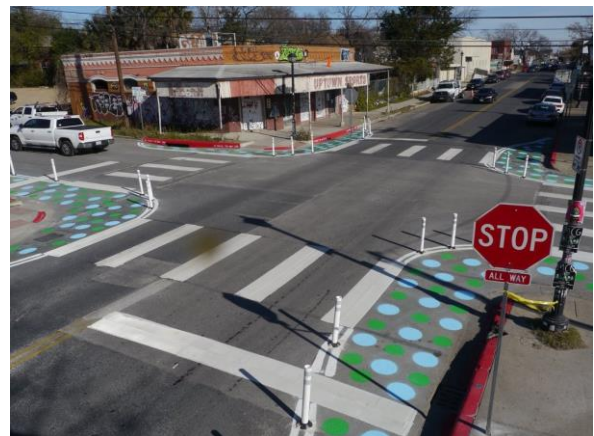
Left: Elements of protected intersections (Source: MassDOT), Right: A tactical approach to narrowed intersections (Source: Austin, Texas)
